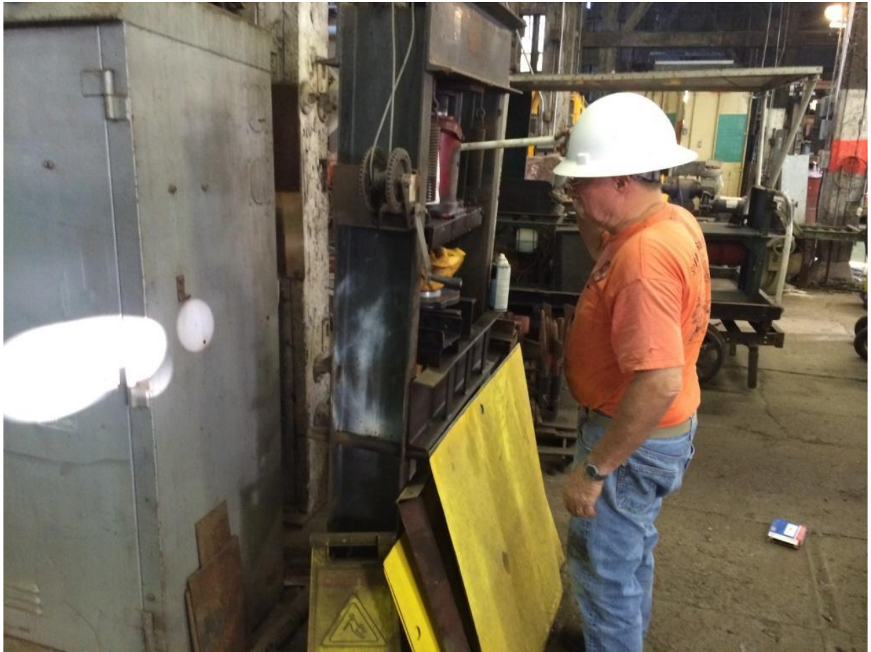
Mike H. pressing the seals into the tamper's new vibration motor
