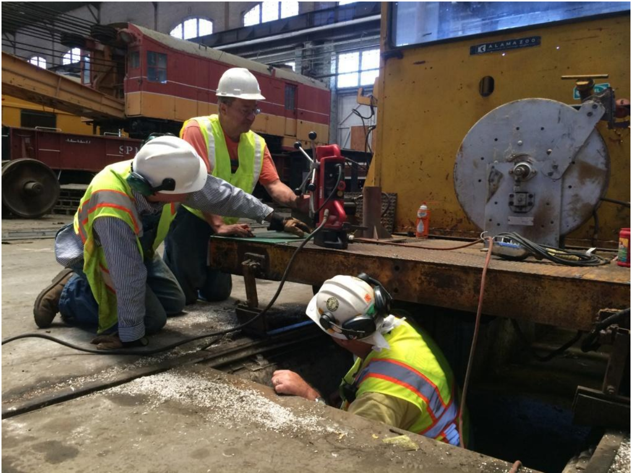
Steve, John, and Mike F. use the mag-drill to install a new deck plate on the Kalamazoo as a base for a small derrick
