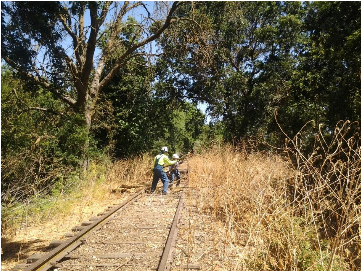
Mike T and Dave clearing the Hood Line
