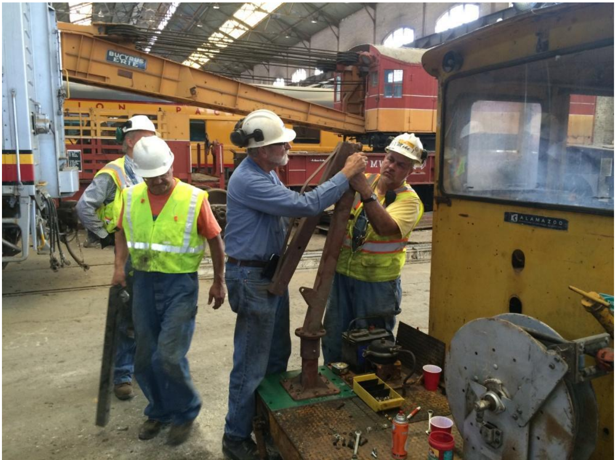
Alan and Mike F. putting the derrick together
