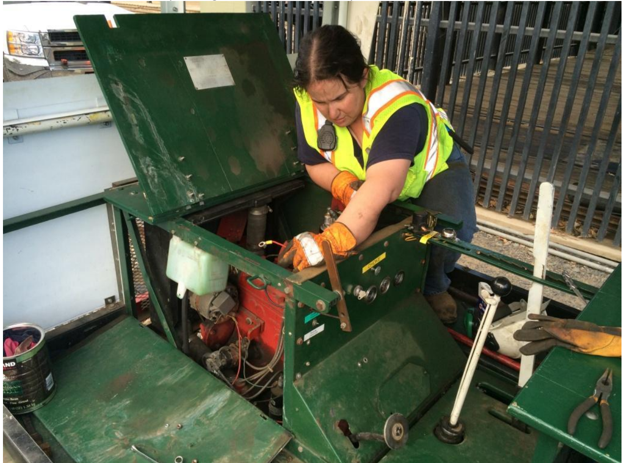
Heather installing the new relay on the MW51 motorcar
